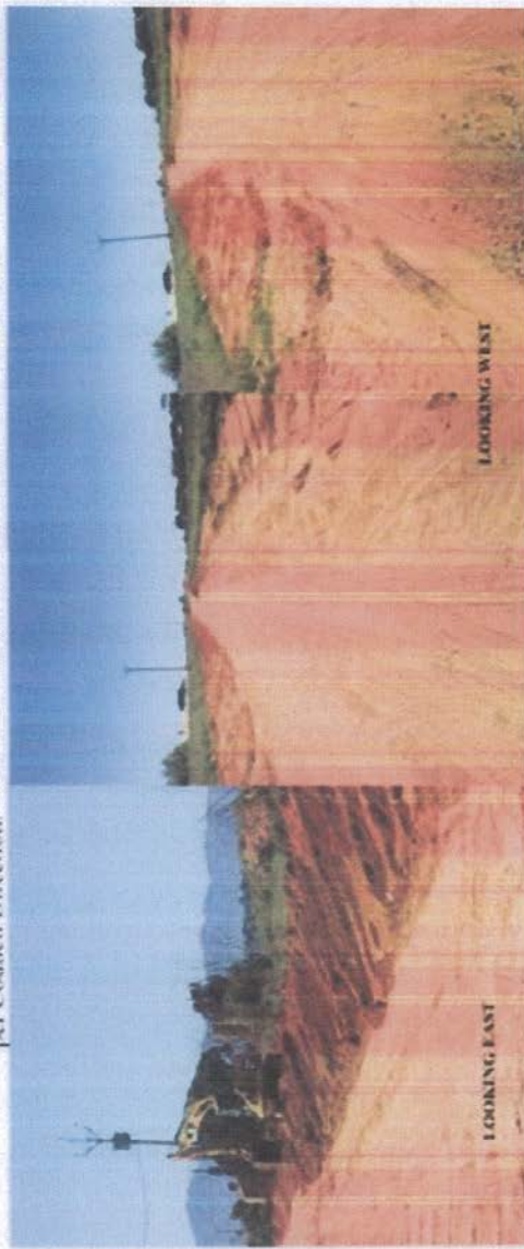
Carosona Road End watermain backfilled where verge used to be, requiring grading and compaction for road surface preparation
